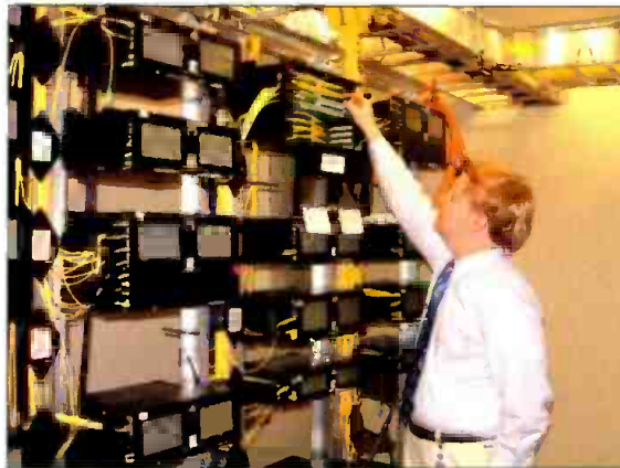
Rick Ackermans, director of engineering for Turner Entertainment Networks, examines the fiber-optic cross-connect facility in Turner's new six-story broadcast facility in Atlanta. The room contains over 600 strands of single-mode fiber and over 300 strands of multimode fiber.
