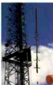
Stacked antenna in Washington, D.C.
